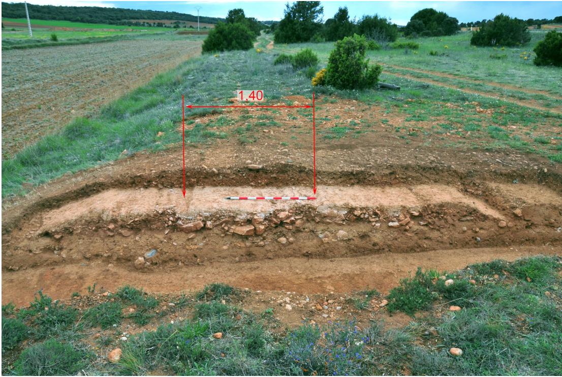
Figure 19, Structure of the Roman road from Numancia to Uxama in Soria, with the tracks of the construction wagons in the intermediate layers of the roadbed. www.viasromanas.net
