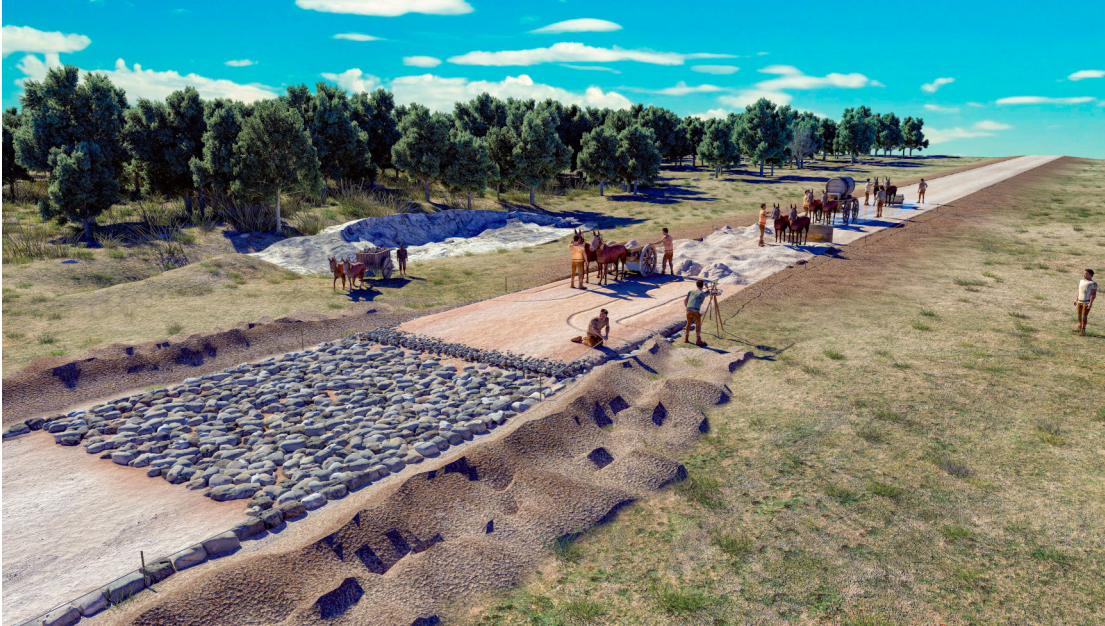
Figure 20, Infographic explaining the construction process of a Roman road and the elements involved
