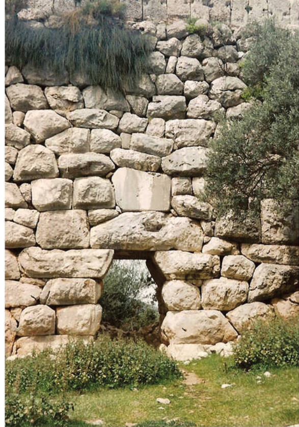
Fig. 15. Cyclopean wall of Delik Kemer siphon, south view. On top conduit stones visible with holes for metal clamps to secure the integrity of the line. The flat stone above the passage bears the inscription (Photo P. KESSENER).
