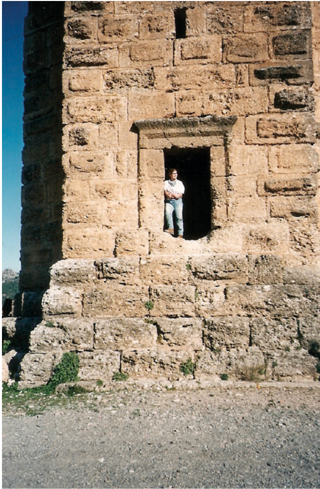
Fig. 28. Aspendos, south hydraulic tower, central part. Entrance to 90 cm wide stone stair way made of stone slabs around central pillar, reaching 15 m high (photo and reconstruction P. KESSENER).
