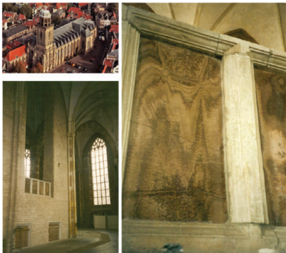
Fig. 4. Choir aisle of the Lebuinus church, Deventer, the Netherlands. Balustrade with sinter slabs (Photo P. KESSENER).
