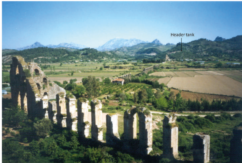
Fig. 26. Aspendos siphon, with remains of two hydraulic towers with sloping ramps, one to the left, one near header tank to the right. View from the Aspendos acropolis (photo P. KESSENER).
