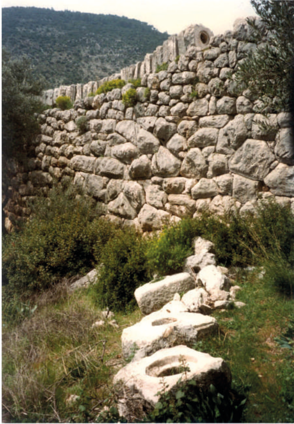
Fig. 14. The 500 m Delik Kemer siphon of the Patara aqueduct (Turkey). Remains of stone conduit built on 10 m high 'Cyclopean wall' (Photo P. KESSENER).
